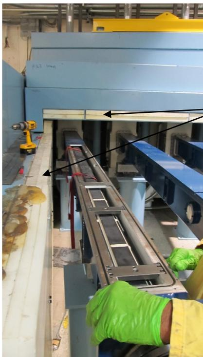
Polyethylene sheets on inside of guide shields in reactor hall C100
