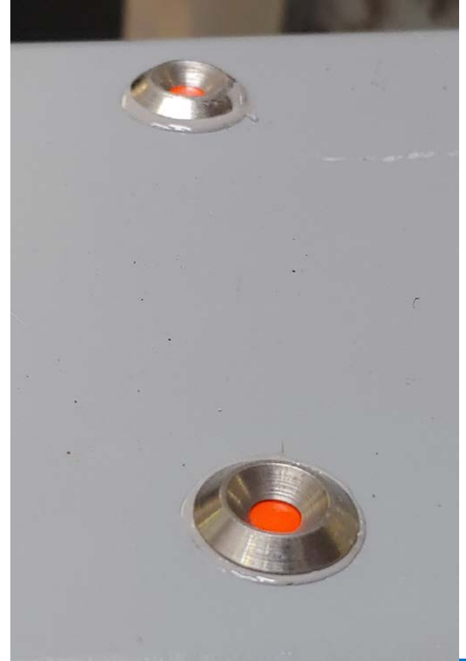
Inexpensive washers for conical-head screws (horizontal surface only).
