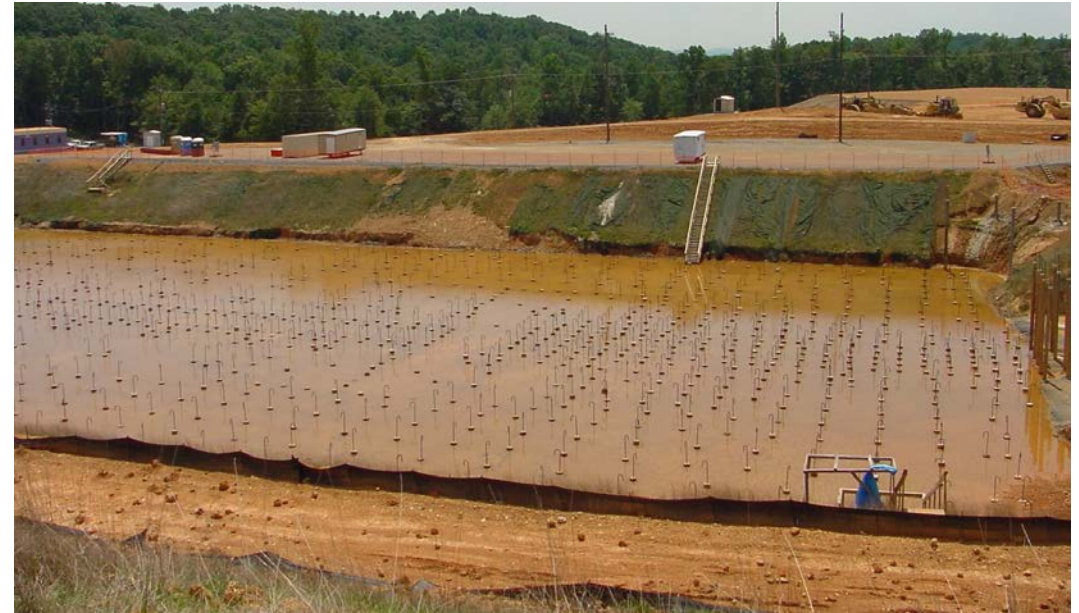
Target building excavation showing typical side slopes
